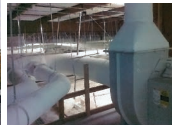
ABOVE Variable speed exhaust fan.
